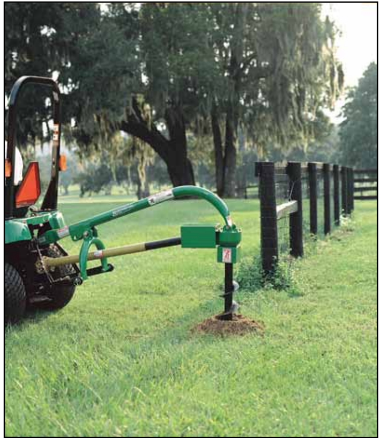
Calling 811 before you begin that outdoor project could help you locate underground services and prevent needless tragedy.
